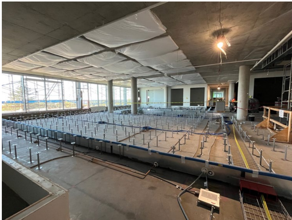
Office level 5 – underfloor and raised floor progress
